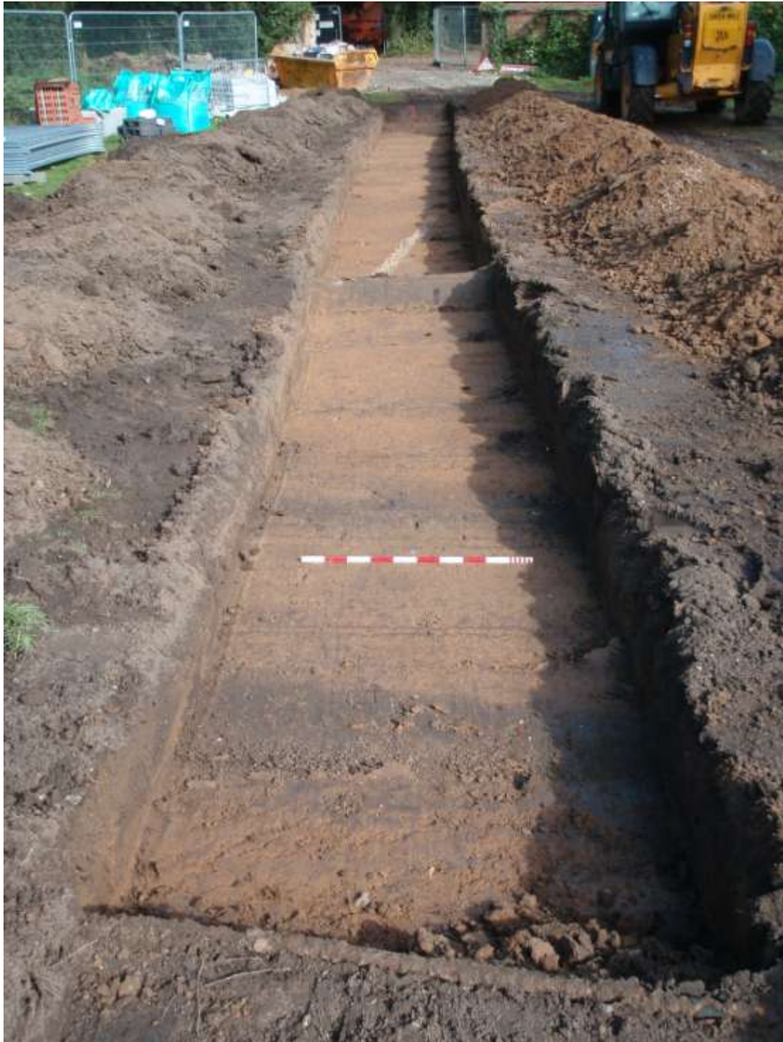
Plate 3. Trench 1 looking north-east, and showing remains of modern pipe runs and field drains
